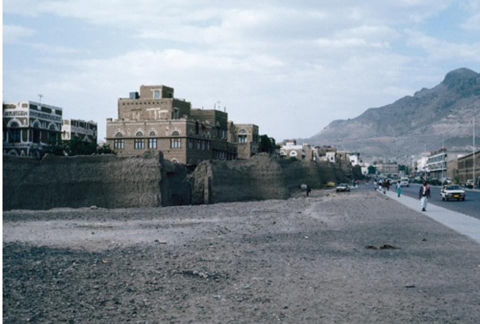
The mud wall around old Sana'a. In arid climates, both buildings and city walls could be kept in good repair even when made of mud.
